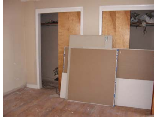
Master bedroom New walls and ceiling Floors to be refinished
