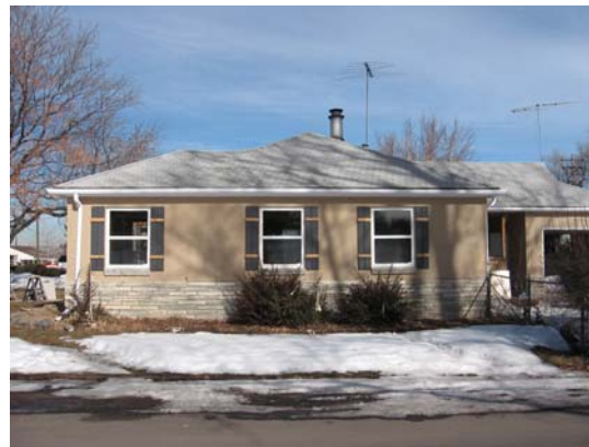
Awnings removed New shutters and paint
