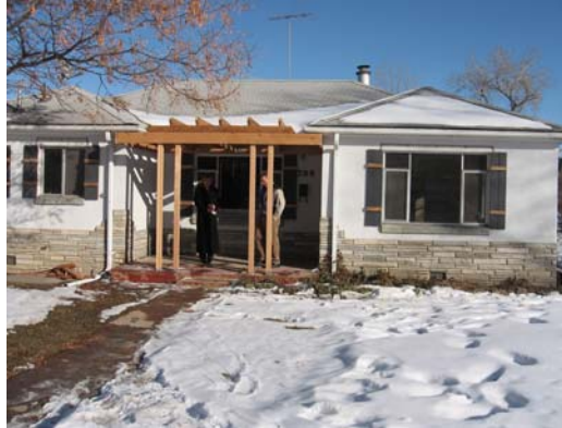
Exterior from W Light comes through new porch cover Old awnings are replaced with decorative shutters, again allowing more light
