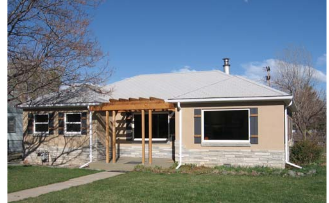
New windows throughout Exterior repainted Old antennas removed
